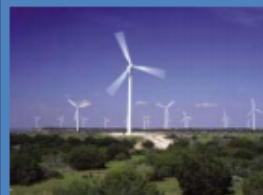
Courtesy of General Electric
